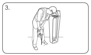
Drill the holes to a depth of 80mm using the 16mm drill bit. Afterwards, take care to ensure the concrete dust is removed from the holes.
